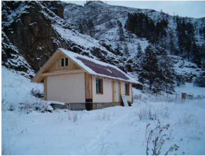
Figure 6: Straw Bale Building in Northern China, Chermal, Altai, Russia. Built by Builders without Borders, The Fund for the 21st Century Altai, 2005
