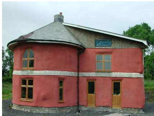
Figure 3: Advantages of Straw. It is simple & cheap. The Spiral House in Ireland, built by Amazon Nails, 2001/2/3
