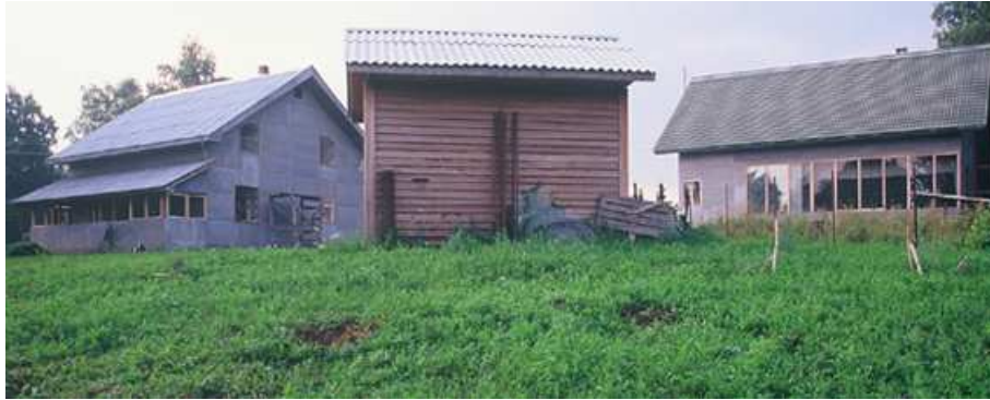
Figure 1.4: View from the south. Vladimir's straw bale house, with a winter garden as a buffer zone on the left, Igor's house with the solar air collector on the right. Sauna in the middle.
